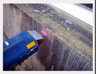
or photons, can discriminate between the soiling and substrate. This allows the conservator to control the level to which the surface is cleaned. Laser cleaning generates very small quantities of waste material (of the order 100 g/m2 for a uniform black approximately 0.1 mm thick on outdoor limestone).
