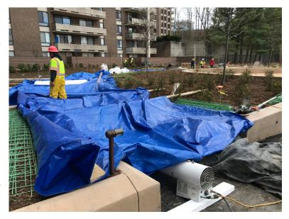
blankets applied to the top surface have minimal impact to the underside of the concrete.
