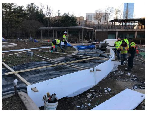
be utilized to evaluate the strength gain of the concrete and whether protections can be removed. When removing protections, if possible they should be removed gradually to reduce thermal shock to the concrete.
